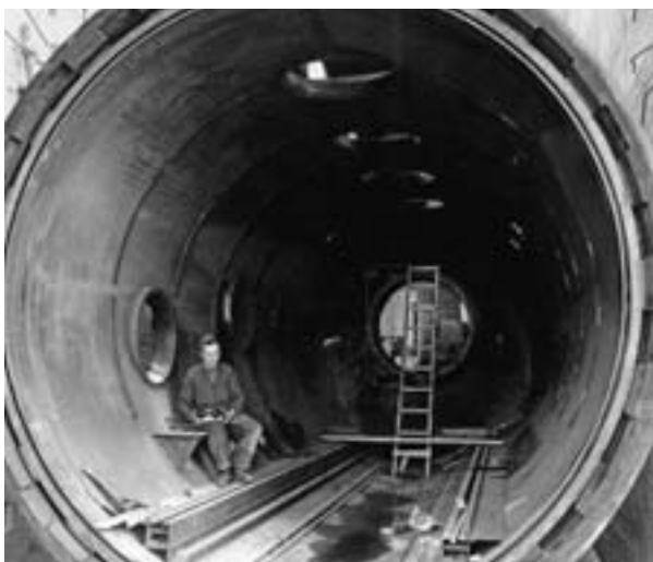
Below left | Construction of the Herbitus low-pressure test facility in Munich, 1943-1944.
